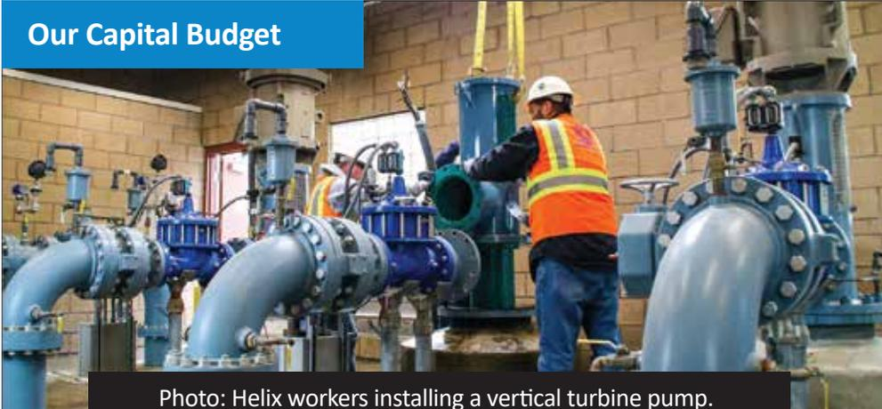
Photo: Helix workers installing a vertical turbine pump.
